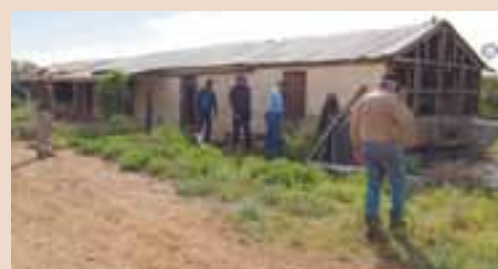
Councilors inspected buildings and infrastructure at Witchelina to see what work needs to be done.
