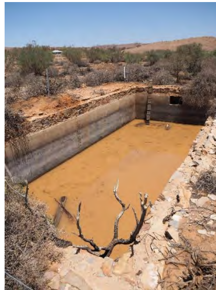
(Below) In-ground tank, half-full of water after summer rain (February 2020). The runged plank at the far end is intended to provide an escape route for any kangaroo falling into the tank when it's dry.
