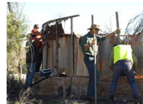
Removing the old water tank at Witchelina.
